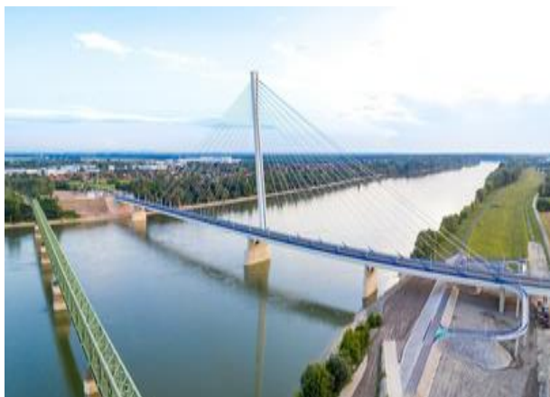
©2014-EU-TMC-0485-W project Connecting Core Network elements in the transport sector: Rhine-Danube Corridor - Komárom-Komarno cross-border bridge
