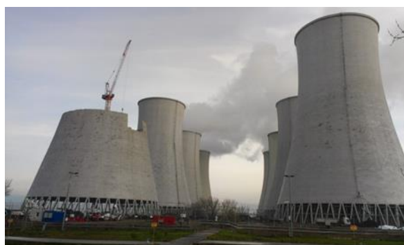
The reactor's cooling circuits have been fully decontaminated
