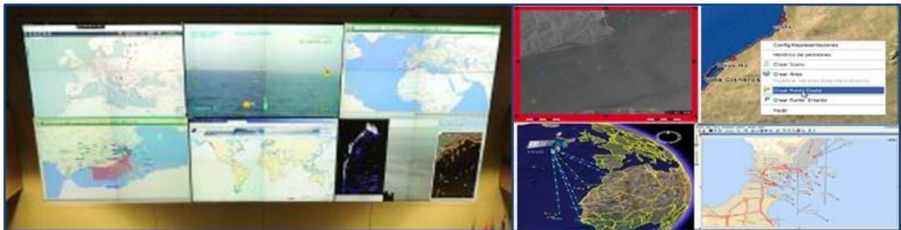
Figure 67: Videowall in the new Operations Room (24 video cubes) (left) compared with the videowall from the original NCC premises (4 cubes) (right)
