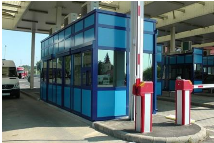
Figure 52: Exterior of the new integrated booths installed at Záhony BCP
