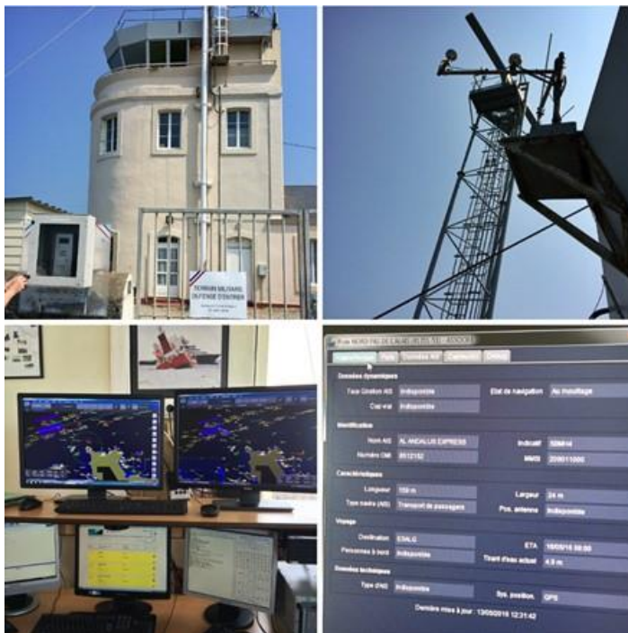
Figure 39: Pictures taken during the field visit at the Semaphore de la Hague, on 13 May 2016. F.L.T.R. and T.T.B: the radar purchased with EBF funding (2) ; the information returned through SPATIONAV (3); the AIS information provided when clicking on a vessel in SPATIONAV System (4).
