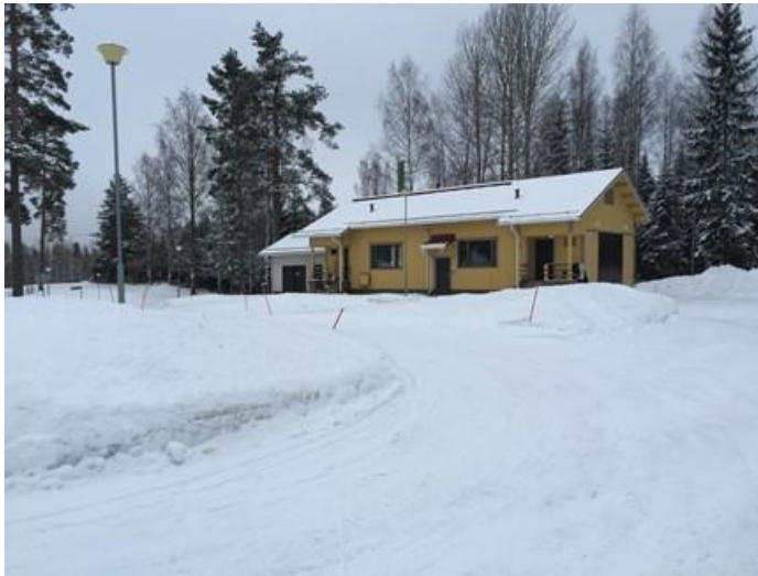
Figure 62: Office facility at the Kolmikanta Border
