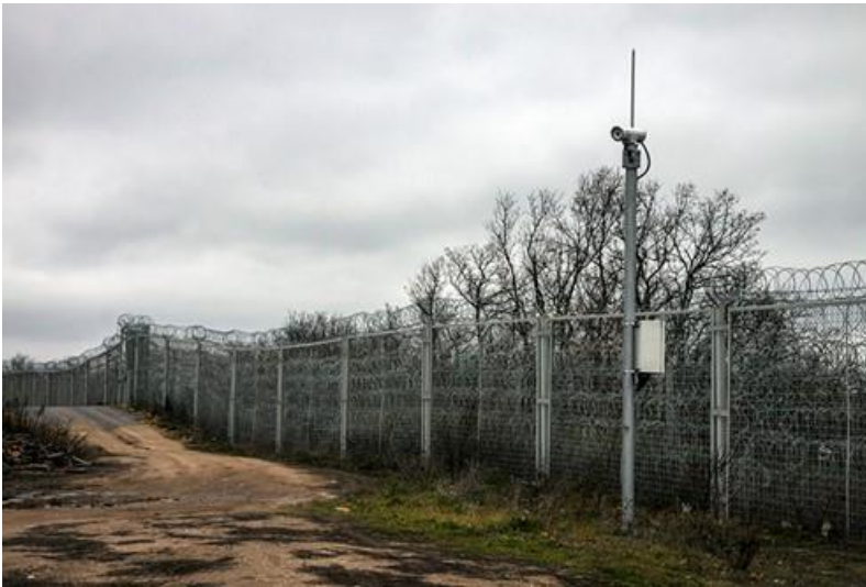
Figure 48: Perimeter surveillance camera and fence
